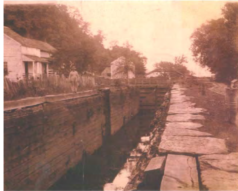
Canal lock 2, Murphy's Hollow. Looking north.
